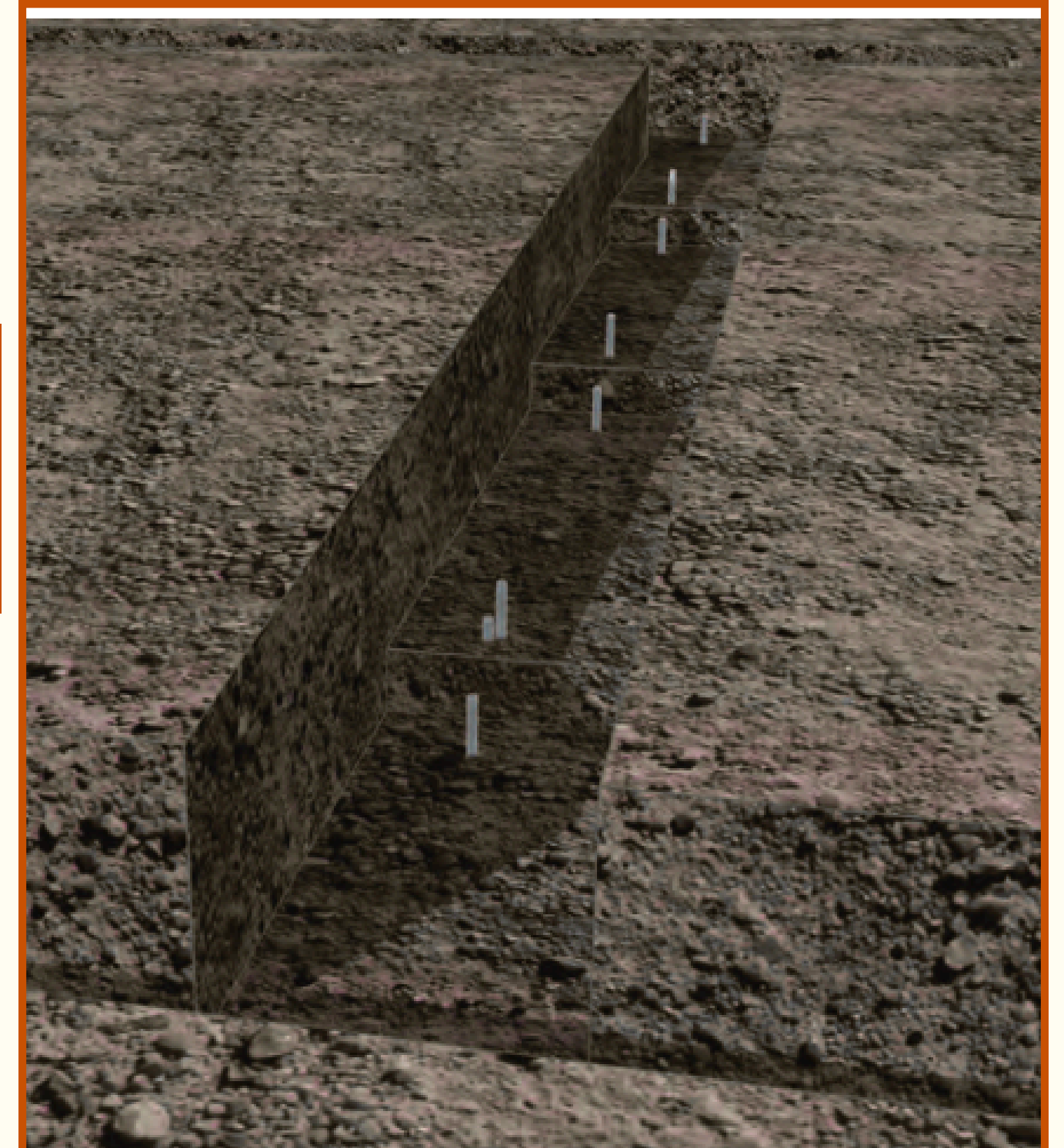
16 Level pegs in position.
