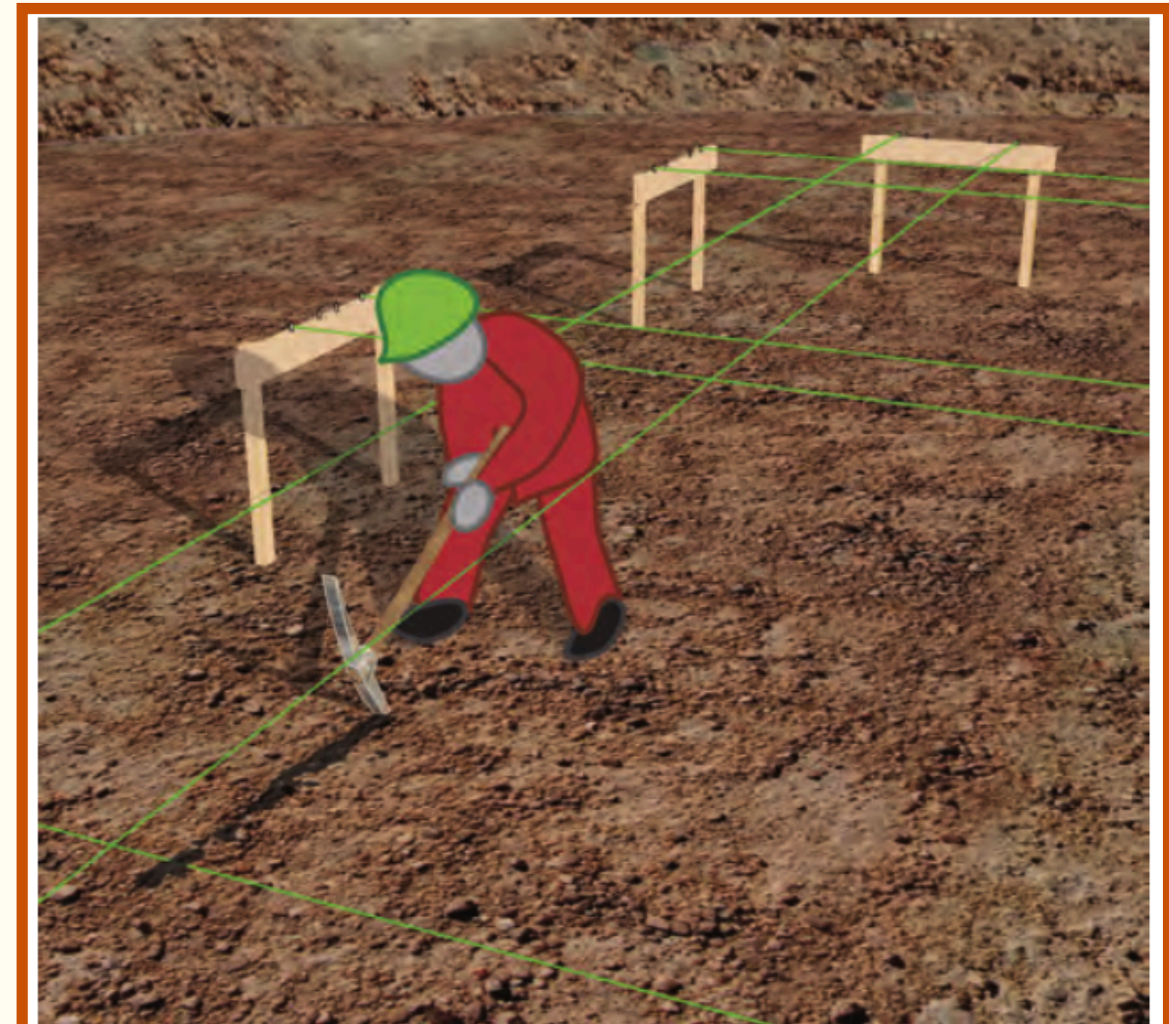
5.11 - The foundation measurements may be transferred to the ground by using a pick as shown
